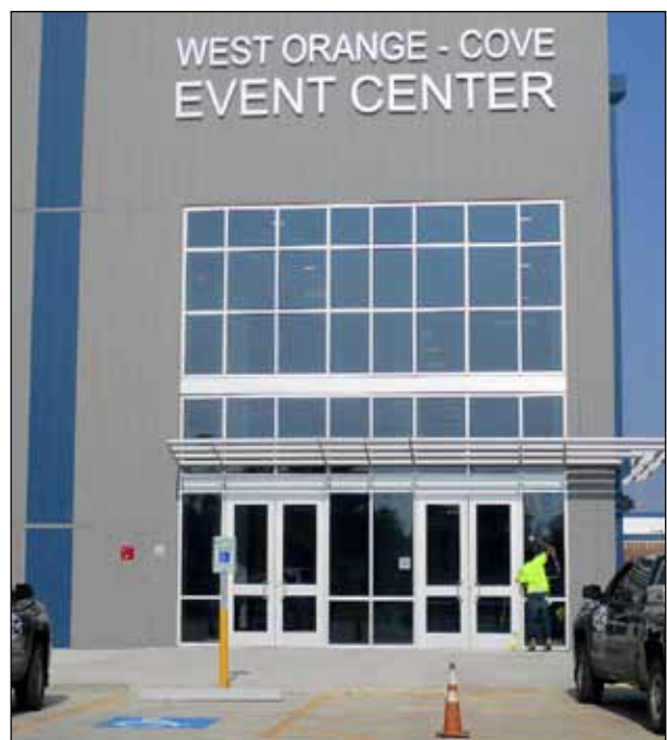
The West Orange-Cove Event Center is 80 percent complete and hosted the graduation ceremony for the 2023 senior class at West Orange-Stark High School on Friday, May 26. RECORD PHOTO: Dan Perrine
