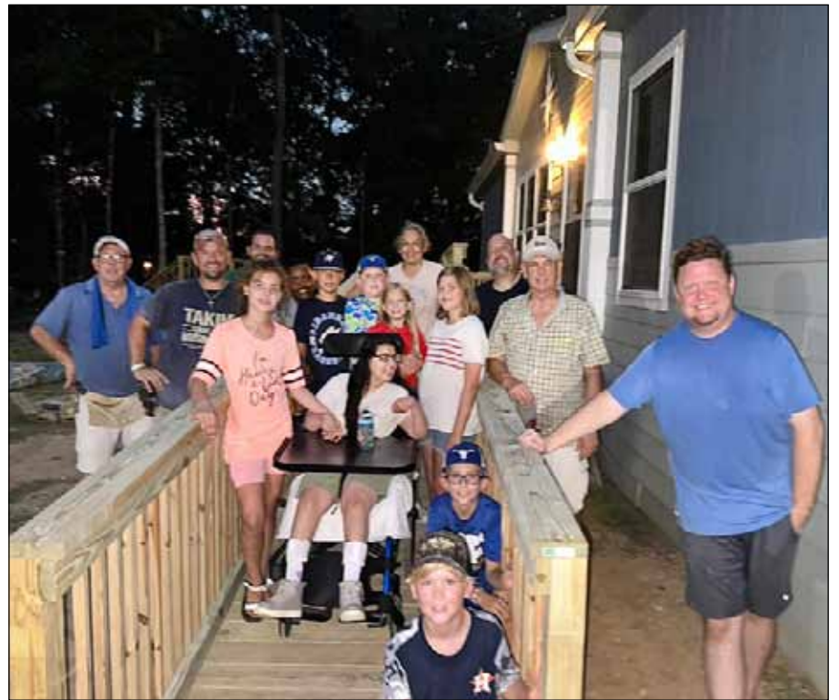
A young woman in a wheelchair now has a professional-style ramp to help her get into her house thanks to a united effort of local volunteers. Workers from the Orange Lions Club, Nehemiah's Vision in Vidor, and Orange County Disaster Rebuild worked in the hot sun and sweltering temperatures Saturday and Sunday to build the ramp. The small, wood frame house previously had a sheet of plywood up some steps. The new ramp is built like a deck with railings and designed in sections to give a safe slope for wheelchair use.
