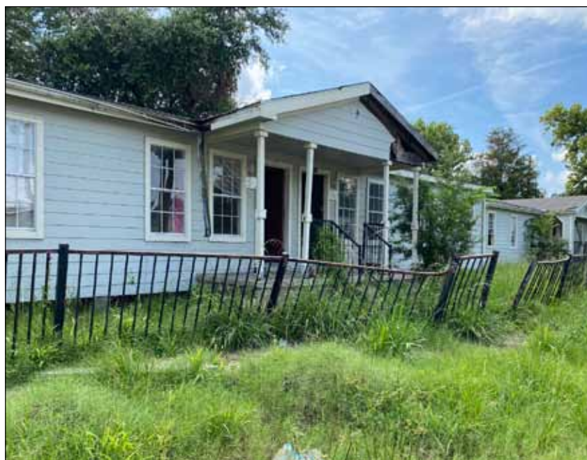
The Orange City Council Tuesday awarded a demolition contract that will cost $145,000 to remove the buildings at what was originally known as Gilmer Homes. The complex between Simmons Drive and First Street in the Old Orange Historic District has been known as Sabine Park Apartments in recent years. It was previously known as The Oaks Apartments. RECORD PHOTO: Margaret Toal
