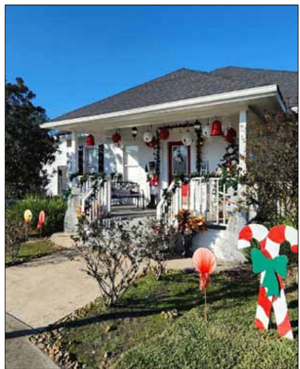
The Bridge City Chamber of Commerce office is decorated for the holiday festivities.
