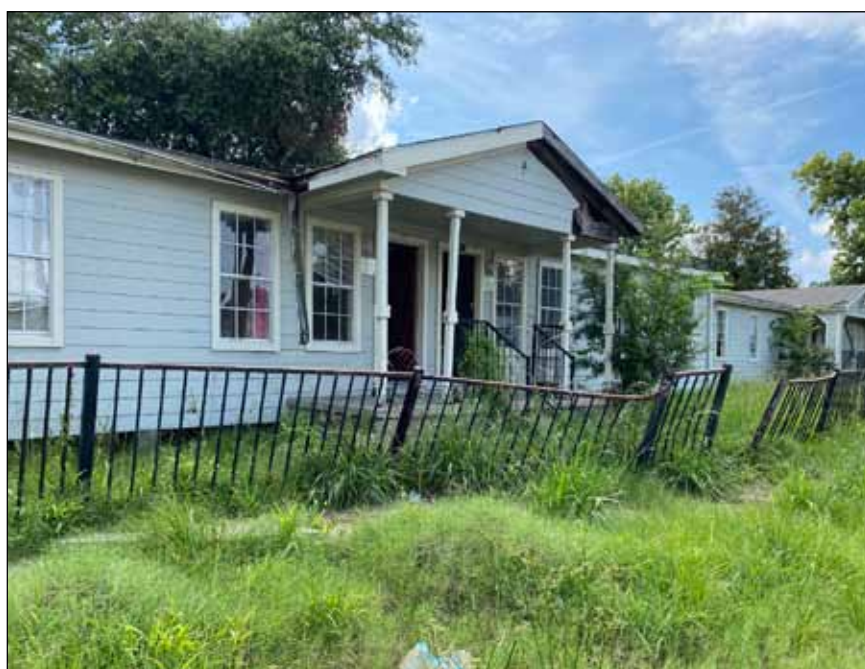
The Orange City Council Tuesday awarded a demolition contract that will cost $145,000 to remove the buildings at what was originally known as Gilmer Homes. The complex between Simmons Drive and First Street in the Old Orange Historic District has been known as Sabine Park Apartments in recent years. It was previously known as The Oaks Apartments. RECORD PHOTO: Margaret Toal
